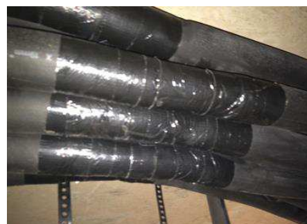
PVC tape wrapped around joints without glue
